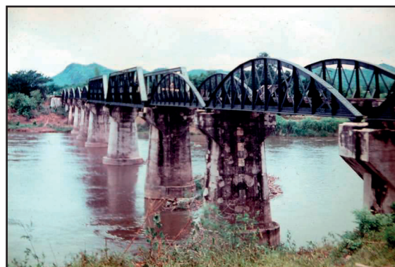
The Kwai Bridge
