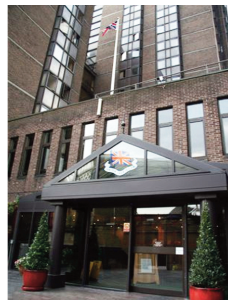
The Front Entrance on Waterloo Road
