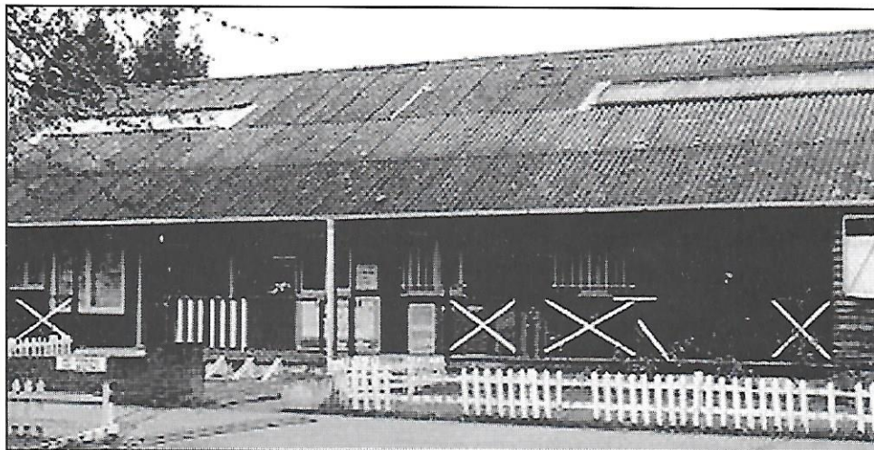
The old Poperinghe Barracks Guardroom
