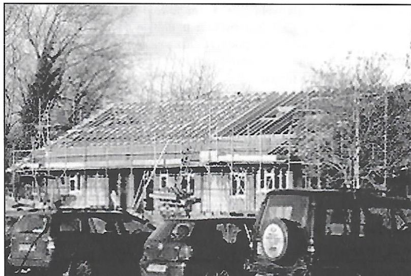
Reconstruction well under way
