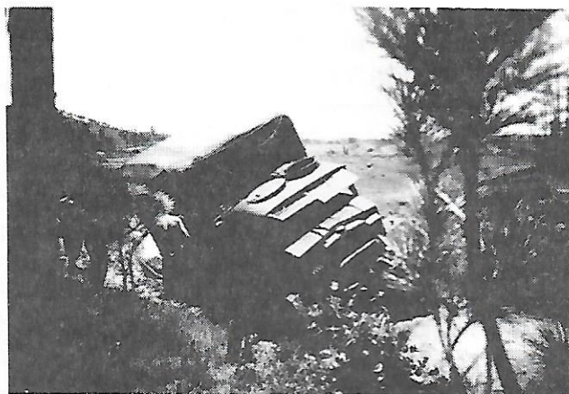
'Karrier', our winch wagon bogged in the ditch.
